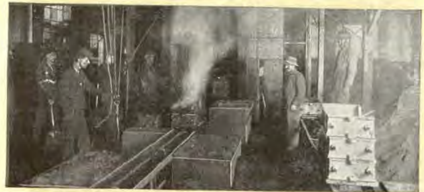
Breaking the Cylinder Moulds
