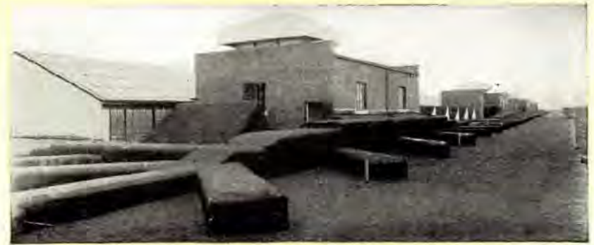
Roof Heating System
