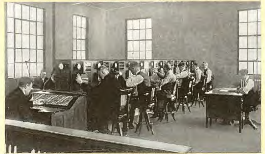
Pyrometers from which the Temperatures of the Furnaces are Regulated
