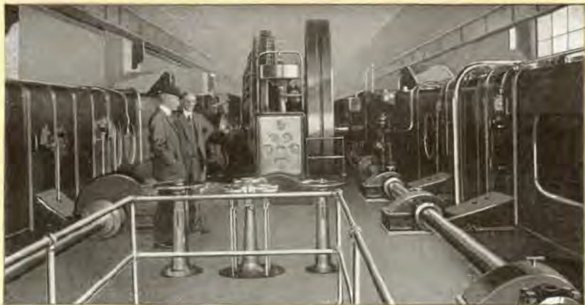
6,000 H. P. Engine—Showing Starting Devices
