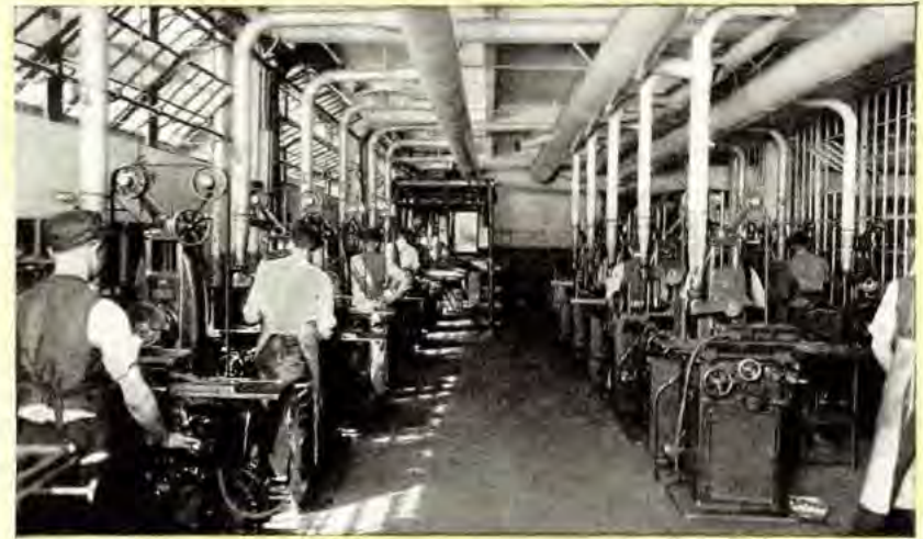
View in Grinding Department, Showing the Suction Pipes Which Remove Emery Dust
