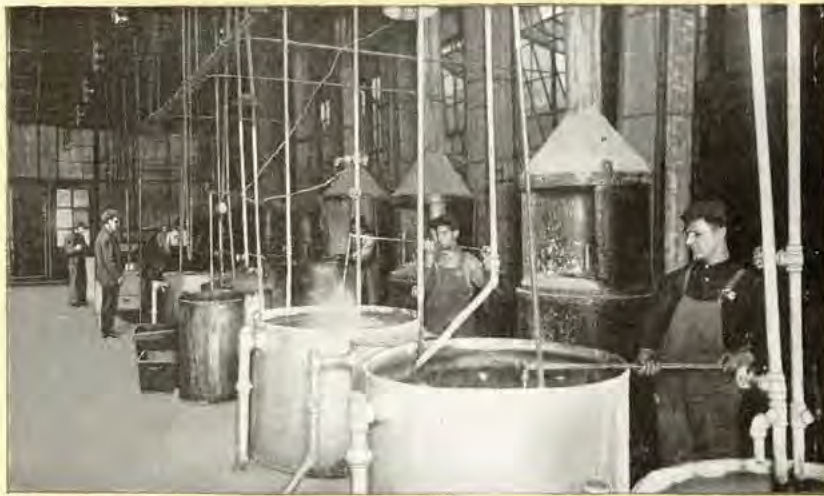
Cyanide Pots and Quenching Tanks
