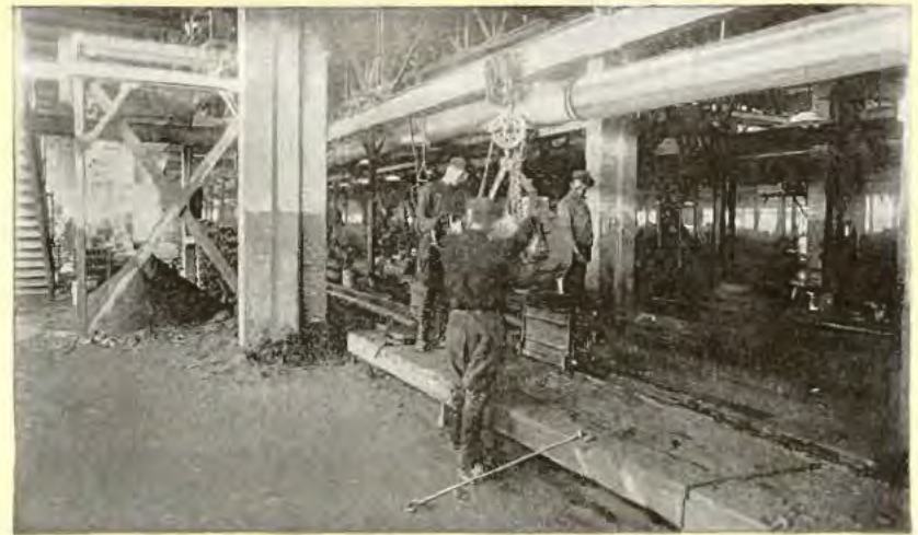
Pouring Molten Iron into Cylinder Moulds
