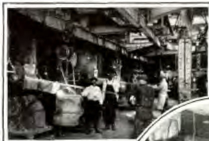
Filling a Ladle at a Cupola.
