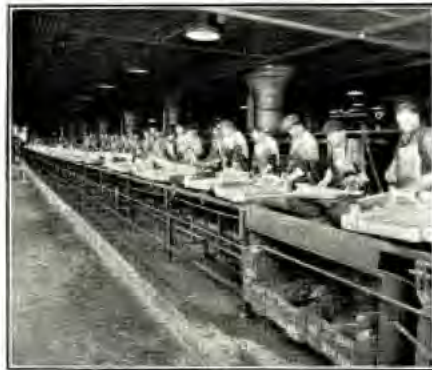
Each Radiator Tested For Leaks
