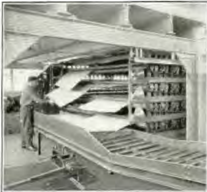
Paper Comes in Large Wet Sheets. Drying is Done in Long Ovens.
