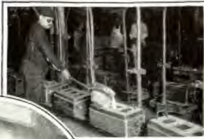
Pouring Castings on a Moving Conveyor.
