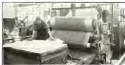
Paper Comes in Large Wet Sheets. Drying is Done in Long Ovens.
