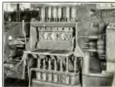
Boring 48 Holes at a Single Operation
