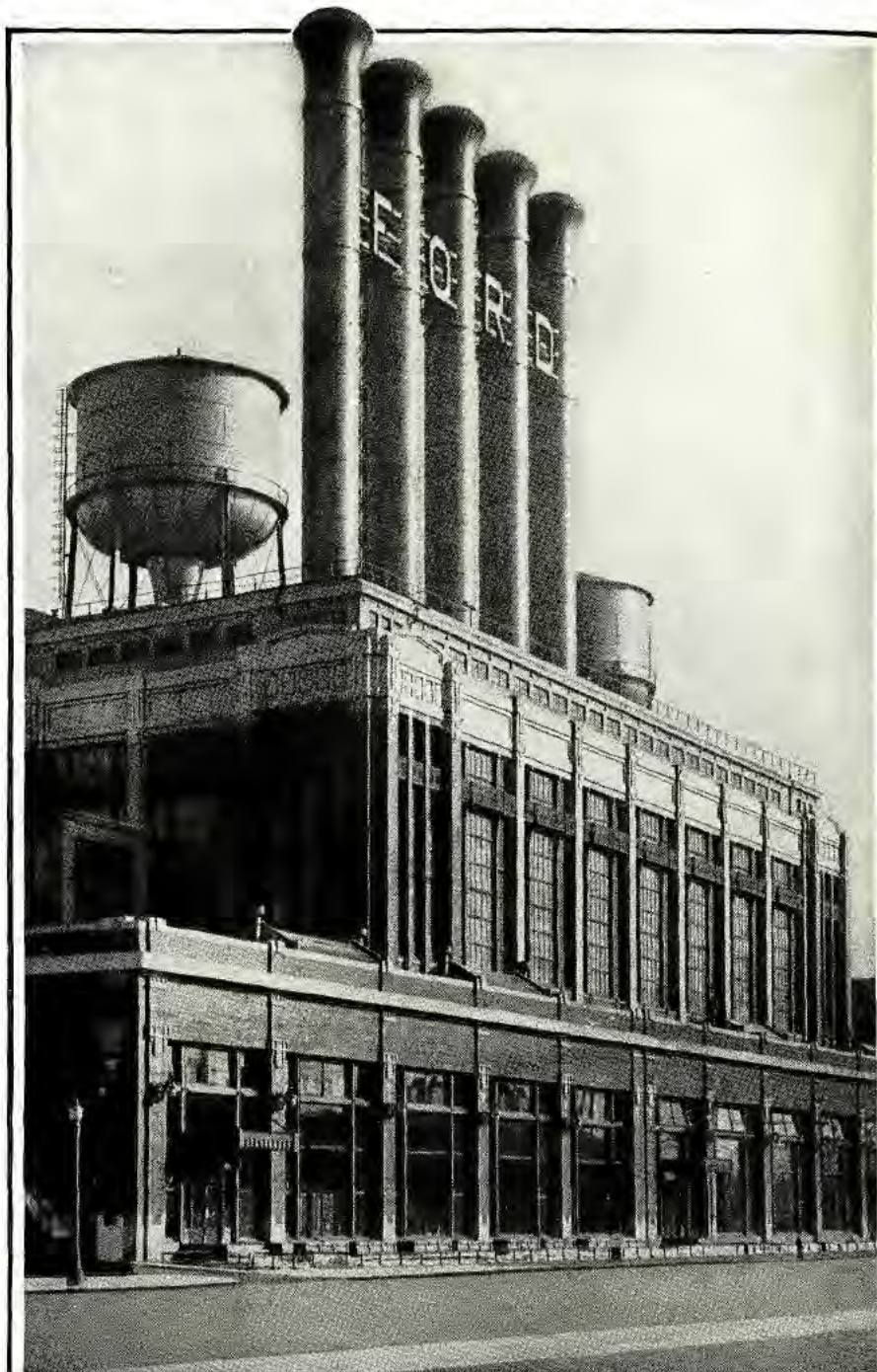
THE HIGHLAND PARK POWER HOUSE
