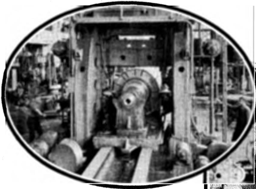
Scene in Highland Park plant showing machining of armature for turbine Generator preparatory to installation in the Twin City plant of the Ford Motor Company.
