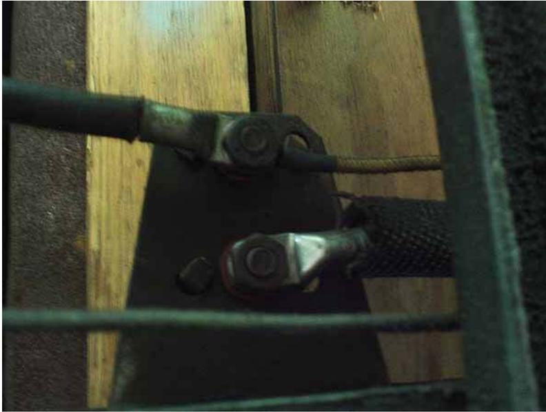
Next, a few inches from the terminal connector, we snip the wire with a pair of diagonal cutters (below).
