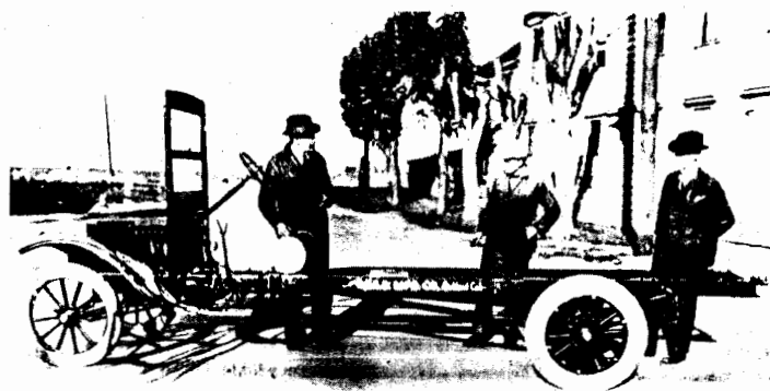
This T-frame extension involved a longer driveshaft and was made by the F. A. B. Manufacturing Co. of Emeryville, CA, later known as FABCO. (Photo courtesy FABCO)
